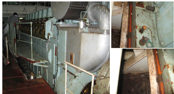
Fig. 6 Installation condition of engine (ship)
