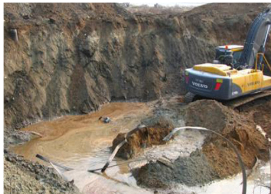
Figure 4. Excavation of contaminated soil in US army base
