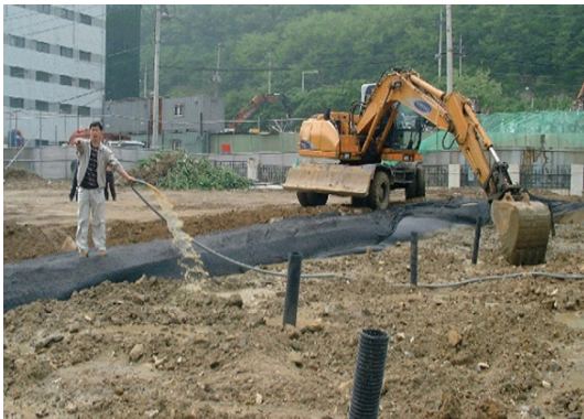
Figure 1. Remediation of Oil spill site
