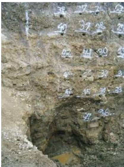
Figure 8. Water inflow at the east side of the hole
