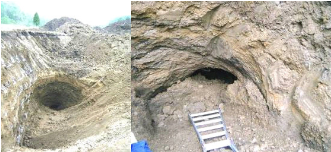
Figure.7. Natural soil pipe due to the internal erosion
