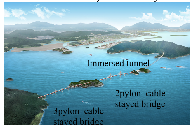
Figure1 1. Overview of Busan-Geoje Fixed Link
