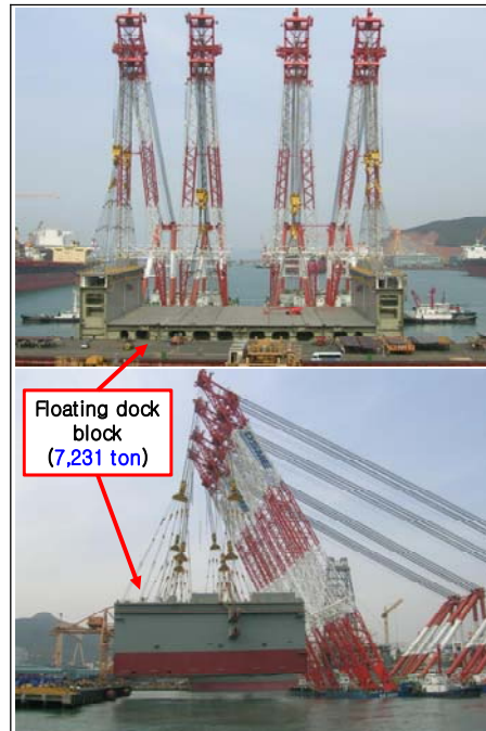
Fig. 21 Example 3: 50Y floating dock block lifting
