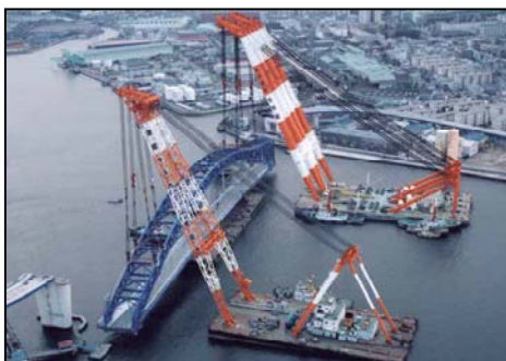
Fig. 3 Erection of arch block by two floating cranes (Ishida 2003)
