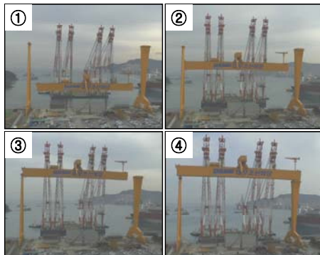
Fig. 19 Example 2: 50Y block lifting
