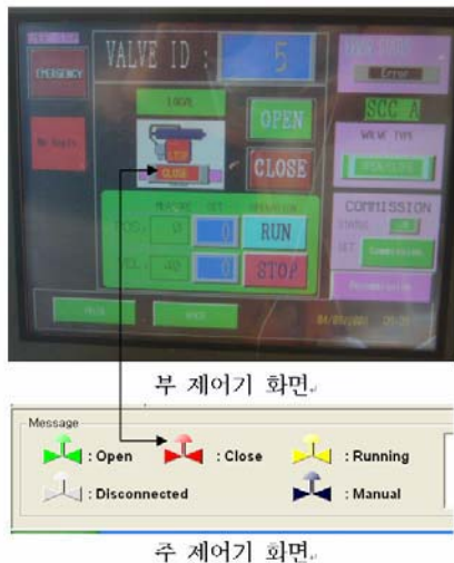
Fig. 11 Display to control and monitor each valve actuator
