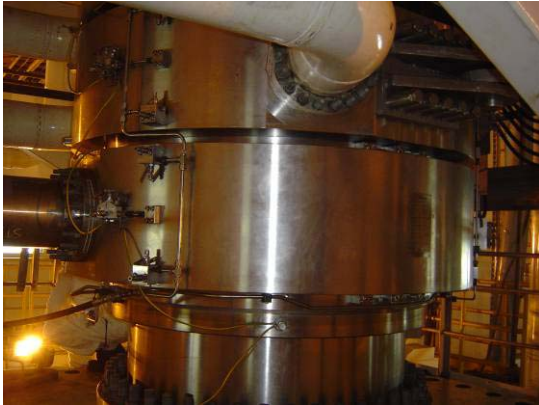
Fig. 11 Picture for Swivel stack after installation
