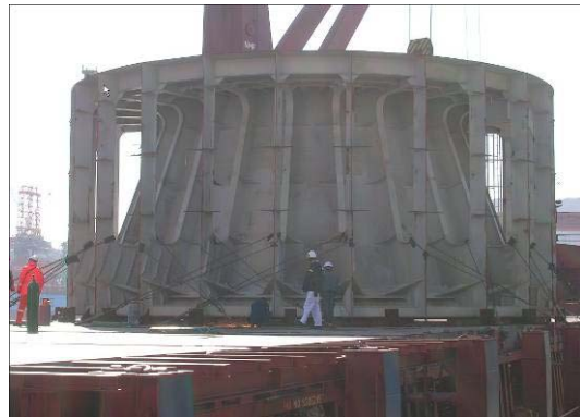
Fig. 5 Picture for construction of MCM
