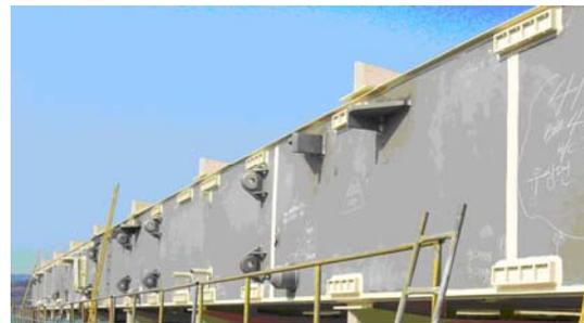
**Fig. 3** Installation of plastic type bearing pad holder on assembly stage
