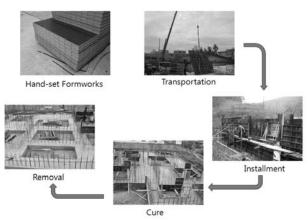
Figure 3. Formwork process breakdown
