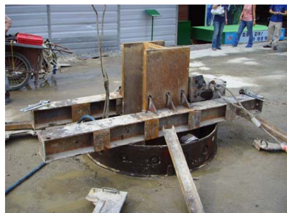
Fig. 3 Pillar Pile Insertion
