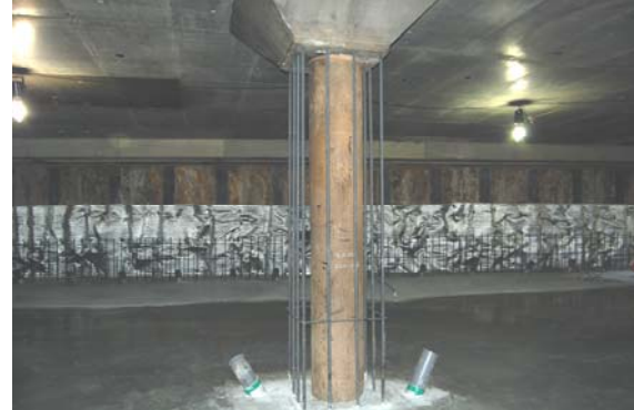
Fig. 11 Pillar Pile Exposed After Excavation
