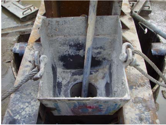
Fig. 4 Tremie Pipe Installation
