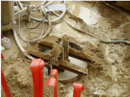
Fig. 12 Wide flange section as a pillar pile
