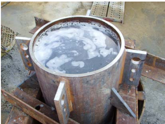
Fig. 13 Circular CFT section as a pillar pile
