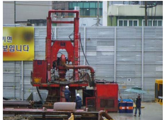
Fig. 2 Boring with RCD Equipment
