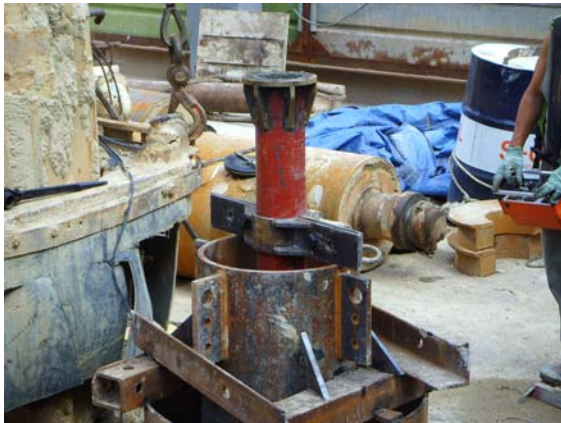
Fig. 9 Installation of Tremie Pipe
