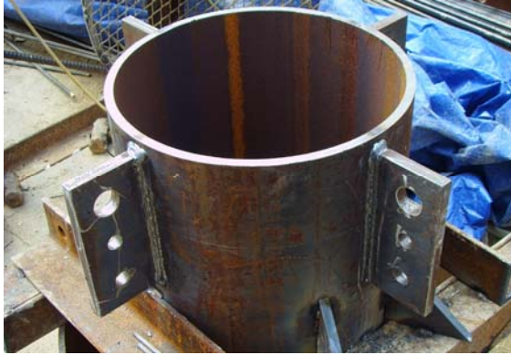
Fig. 8 Pillar Pile Insertion
