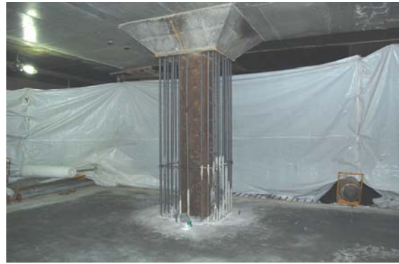
Fig. 6 Pillar Pile Having Been Exposed After Excavation
