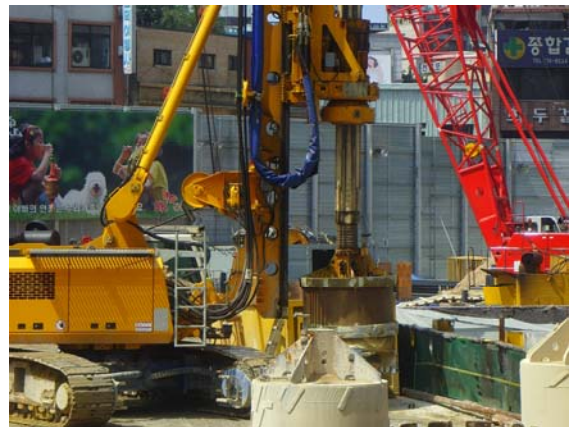
Fig. 7 Boring with PRD Equipment
