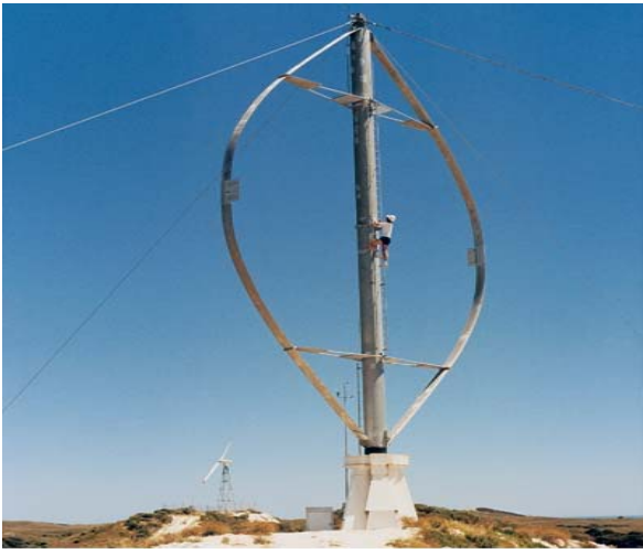
Figure1. Darrieus Wind Turbine
