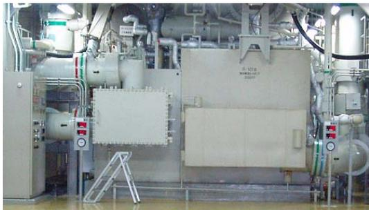
Fig.2 Photo of seawater heat pump
