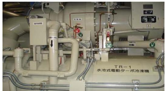
Fig.11 Photo of turbo refrigerator
