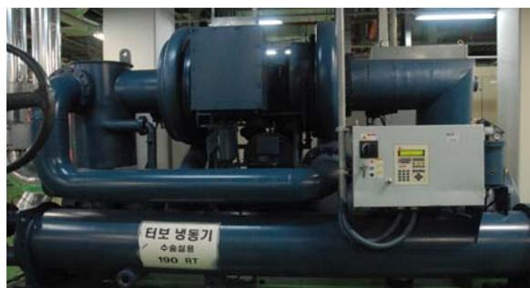
Fig. 1 Picture of Centrifugal water chiller
