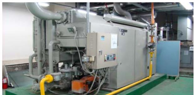
Fig. 3 Picture of Absorption system
