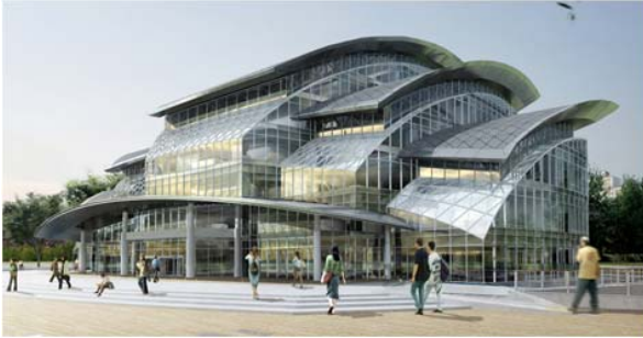
Fig. 1 Air-view of the evaluated building
