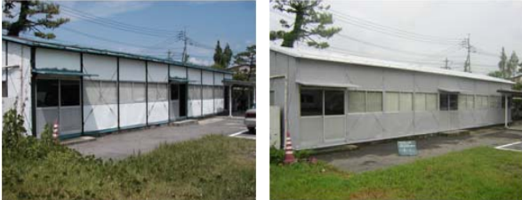
Fig. 17 Complex building in Saga Japan before and after the heat exchanging paint applied
