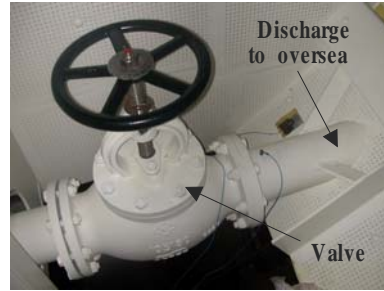
(a) Construction of the discharge pipe and valve
