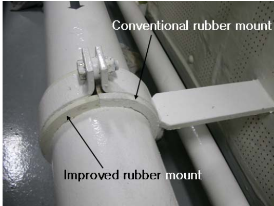
(e) Construction of Rubber Mount
