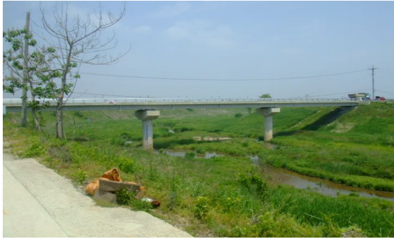
Fig. 2 WPC girder bridge
