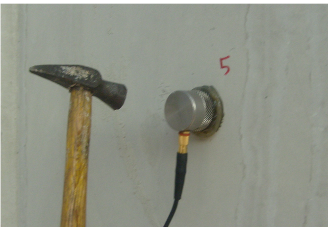
Fig. 4 Concrete thickness measurement using impact resonance test
