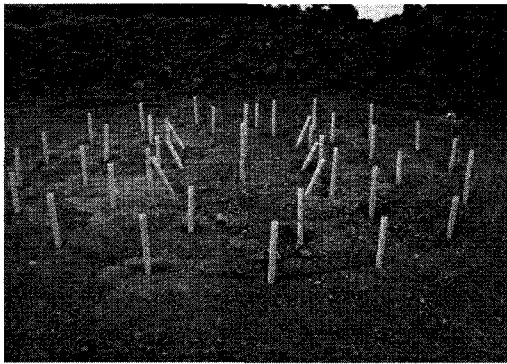
(b) Drilling pattern of V-cut
