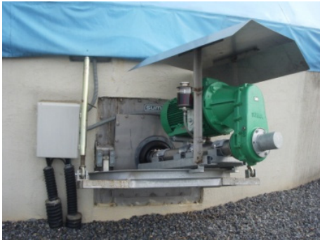
Fig. 3 The agitator of inclined type(30° sealing plate version)
