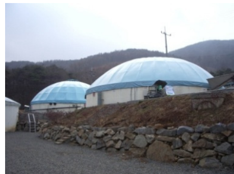
Fig. 2 The anaerobic digester for treatment of piggery wastewater and biogas production
