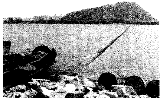
Fig. 1. Sediment-Inflow Protection Weir
