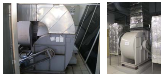
(a) Building A
