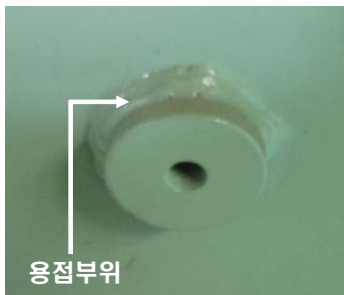
(a) Full Welding type Outer Hinge
