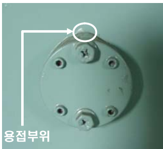
(b) local Welding type Outer Hinge
