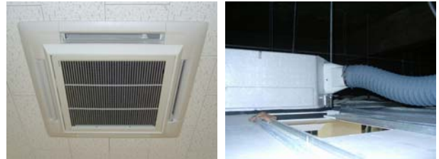
(b) After installation of unit, duct etc.
