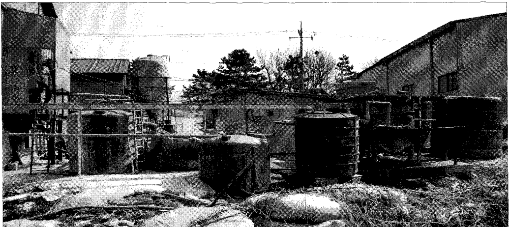
Fig. 1. ECO Pilot Plant.
