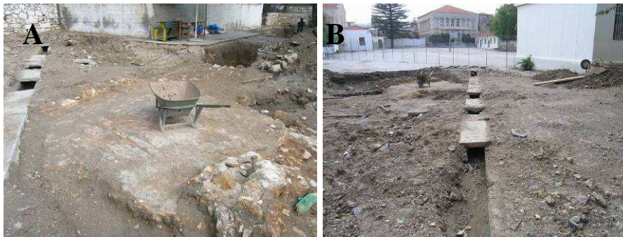
Fig 6. A) Excavated structure at the north of the Turkish school area related with the anomaly T10. B) Modern drainage related with the anomaly T1.
