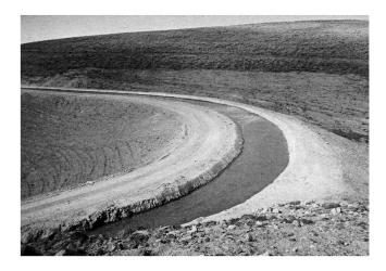
The selected less weathered material was specified in the expectation that the surface would "self armour" itself more quickly than if no attempt was made to select coarser material. Each transition from cut section to fill section was approximately 10 metres long and not necessarily coincident on either side of the canal. Despite the versatility of 12D's conditional profile feature the chainage of each transition had to be set manually after each change in centreline location.
