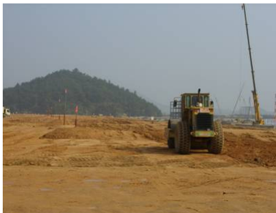
④ Embankment-2, 0.7m
