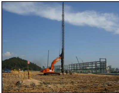
⑤ Installation of PVD
