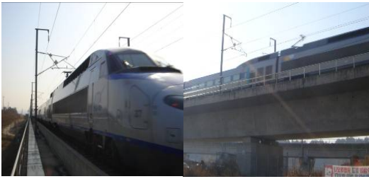
Fig. 3 Photo for the overhead contact line monitoring system installed at Yeonje bridge in Korean high-speed line.
