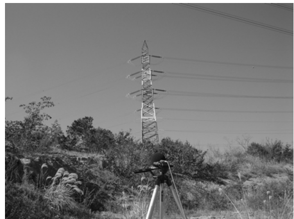
Fig 6. Transmission Power Line Noise for 765kV
