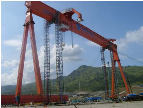
Fig. 1 Photograph for hoisting a large crane
