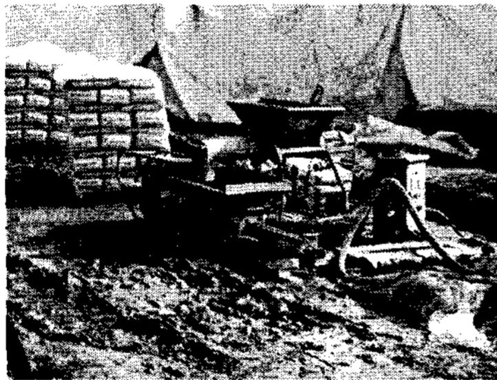
Fig. 6 Injection of Cement Grout
