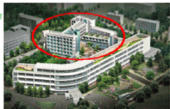
Fig. 1 Building of the ground source heat pump installed.
