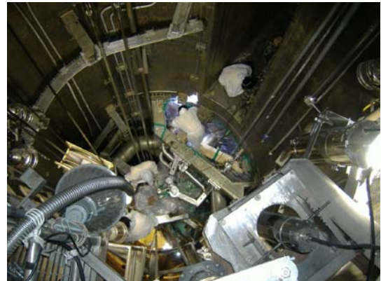
Fig 7 Installation of In Pile Section
