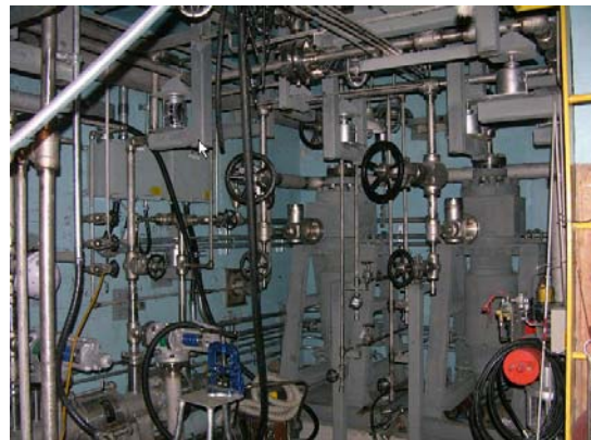
Fig. 5 Construction of Room #1
