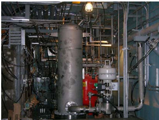
Fig. 6 Construction of Room #2
