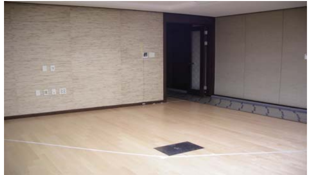
[Fig.9] Measuring view of indoor and floor surface temperature
