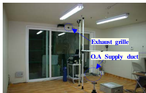
(b) Air incoming part and exhaust grille
