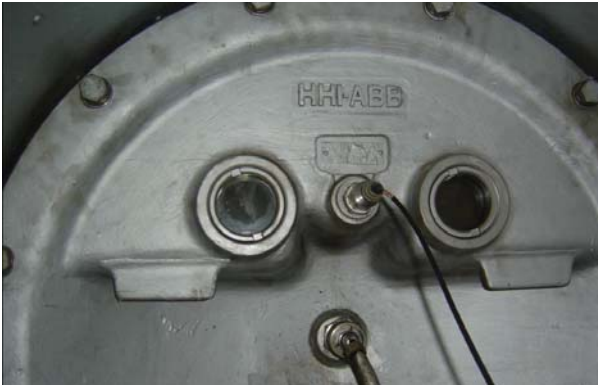
Fig. 8 Vibration measurement at blower side of turbocharger for two stroke low speed diesel engine
