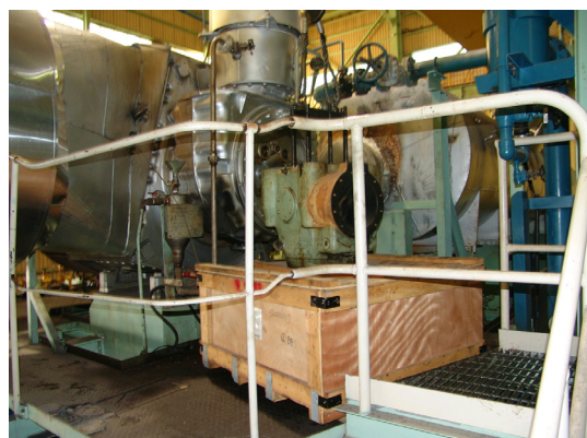
Fig 13. View of adding mass for engine vibration test
