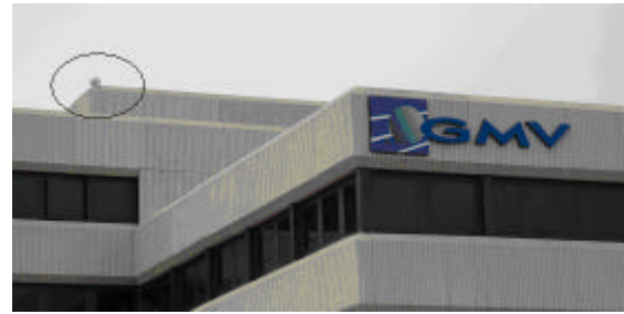
Figure 3. MAGIC Reference Station installation
