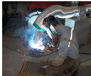
Fig. 6 Welding of bell-mouth
