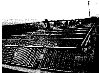
Fig.1 Cheju seasonal storage system with 50 modules of double skin solar collectors.
