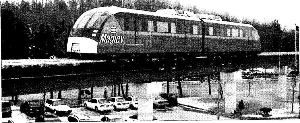
Fig. 1. Rotem Maglev running over an elevated guideway
