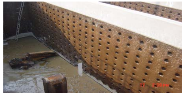
Fig. 1 The existing rectification wall with holes
