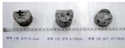
Figure 2. Core boring concrete samples.
