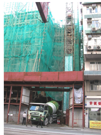
Figure 3. Photo of the Hoist & Barrow concreting site
