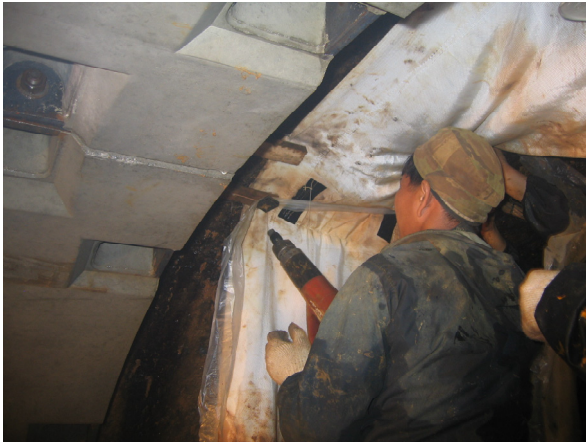
Figure 10. Bullflex Installation
