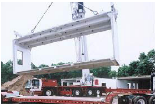
Figure 4. On-site Assembly of prefabricated panels
