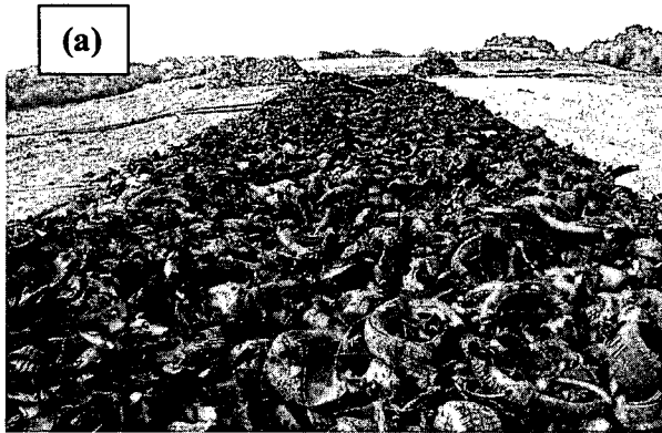
Figure 2: Photograph of the field-scale permeable blankets constructed at an MSW landfill made up of recycled (a) shredded tires; and (b) crushed glass.
