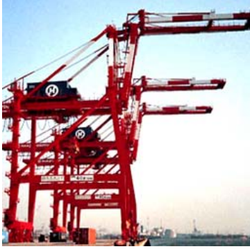
Fig. 1 Articulation type container cranes in Kaoshiung, Taiwan
