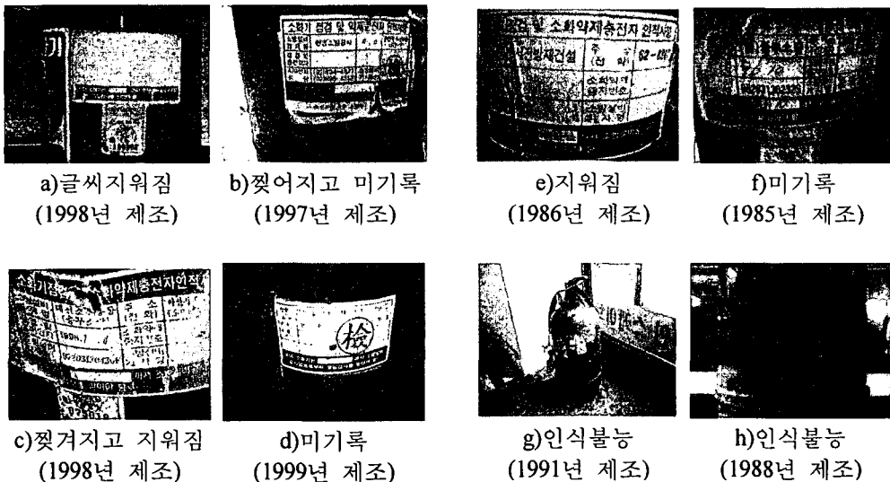
Fig. 5. Damaged or erased stickers
